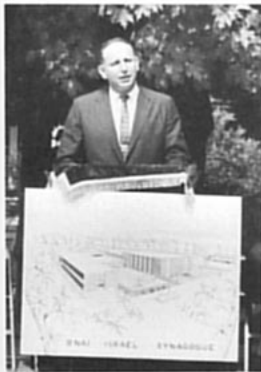
Paul Goodwin, president, presides at the ground breaking July 19, 1959.
